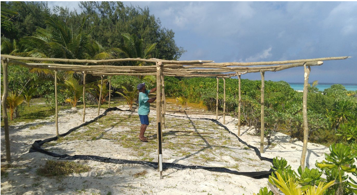
Figure 35: Due south full sun hatchery in construction
